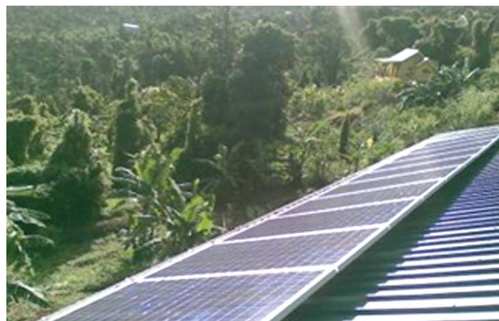
Image 5: Stand-alone system, 1.8kWp Courtesy of www.grensol.com
