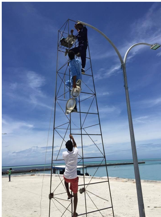
Figure 5: Installation of Energy saving lights
