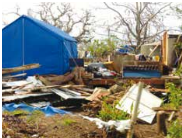
Figure 7.2 Immediate relief shelter provided after Cyclone Ian (credit: MIA)
